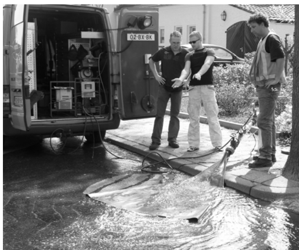
Fig. 2. Flushing of a distribution main
