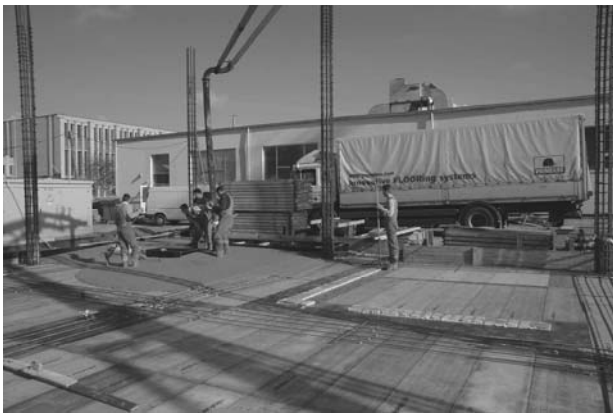
Fig.1. Floor concreting in Daugavpils, Latvia.
