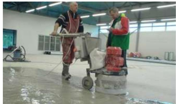
Fig. 2. Rigid polishing of concrete floor surface
