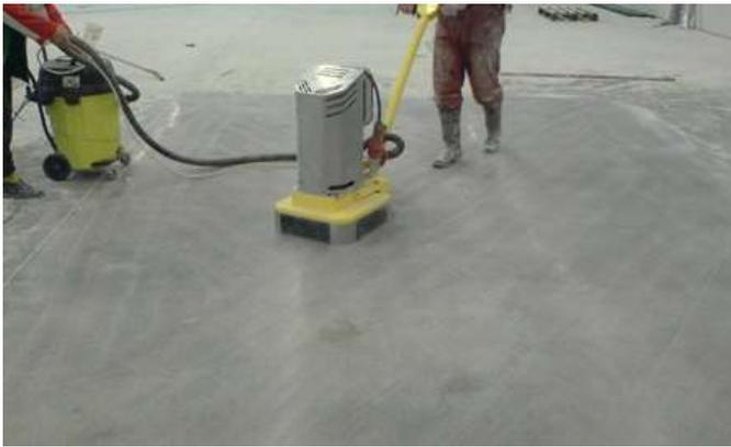
Fig. 3. Floor polishing and grinding
