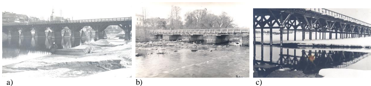
Fig. 6) Examples of the timber piers in Latvia until 1941: a) Bridge over the river Gauja in Valmiera; b) Timber bridge; c) Bridge over the river Pedele in Valka
