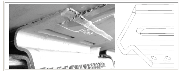
Fig. 10. Crack in transversal seam of the pad on wagon and in the model
