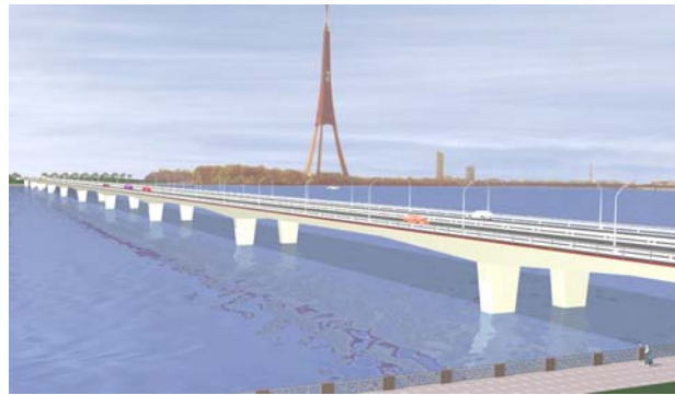
Fig.14. Cross section and visual impression of continuous box girder bridge
