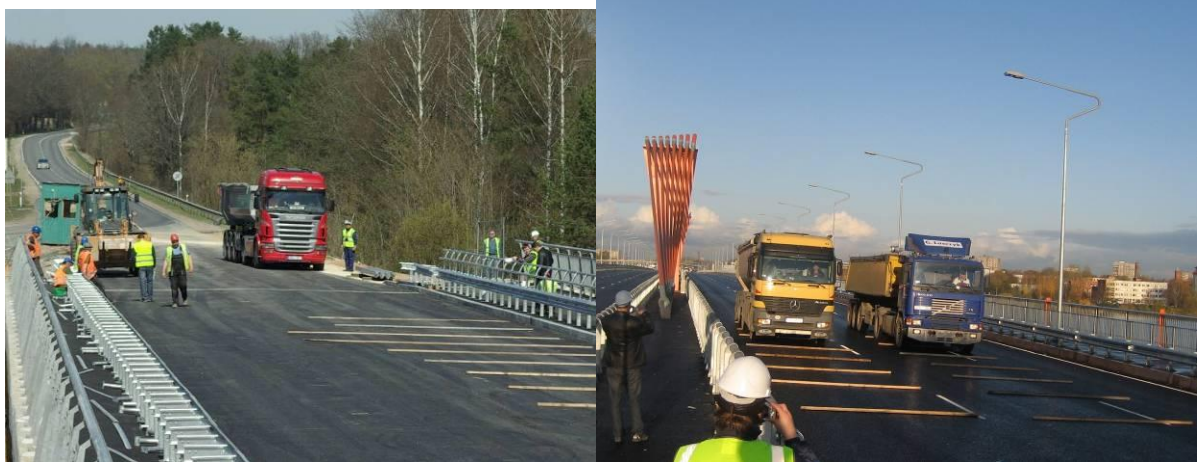
Fig.5 Dynamic loading of Murjani and the new Dienvidu bridges
