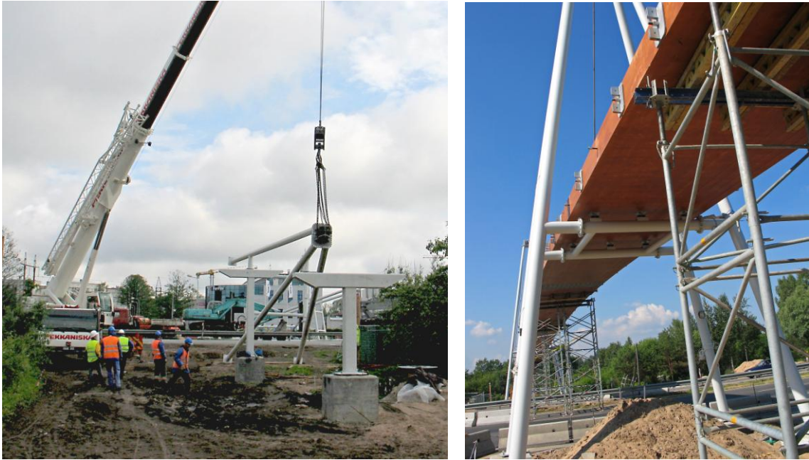
Fig. 4 Placement of the pylon and temporary supports for the deck
