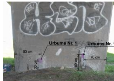
Fig. 5. Core sampling from the ramp No.8 pier.
