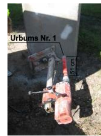
Fig. 6. Ramp No.5 pier and sampling location.
