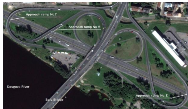
Fig. 1. The right-side approach ramps complex of the Salu Bridge over the Daugava River.
