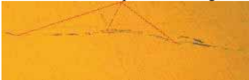
Fig. 1. Lack of fusion of base metal and weld metal
