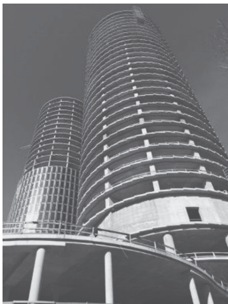
Fig. 1. Multifunctional complex “Z-Towers” during construction
