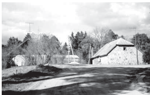
Figure 10. The group of mill buildings (Photo by Zilgalvis)
