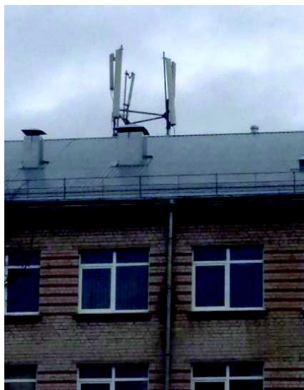
Figure 6. The source of radio frequency exposure for the highest exposure case –a cell phone base station on the adjacent building.
