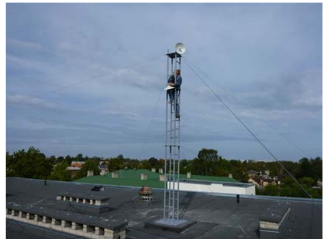
Figure 2. 5GHz networks bridges used to create the base network
