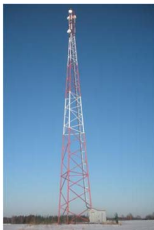
Figure 1. Mast of the tower type
