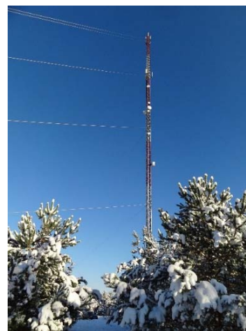
Figure 2. Mast of the guyed type
